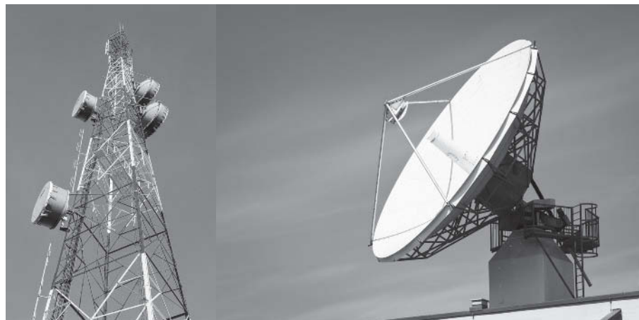
(a) A microwave relay tower
